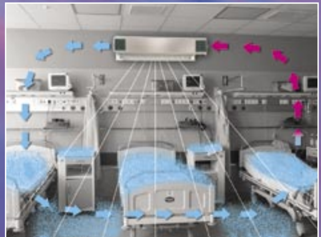
Process of the air treatment with the use of internal and external radiators (air and surfaces)
